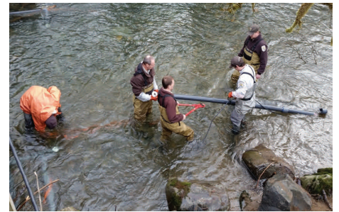
Kyle Hanson, Richard Glenn, Will Simpson, Doug Peterson, and Ben Kennedy repairing storm damaged remote monitoring antenna array in Abernathy Creek. Photo credit: K. Hawke.
